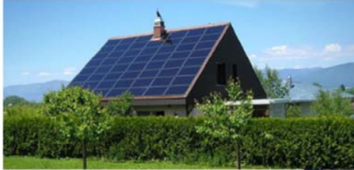
Residential photovoltaic installations - Germany
