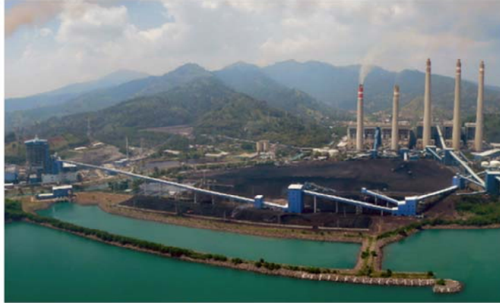
Suralaya coal-fired power station (4,025MW) - Indonesia
