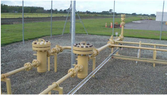
Figure 3 - Filters at the start of two metering 'streams' on a transmission system delivery point (source: Vector Gas Transmission Asset Management Plan 2013)
