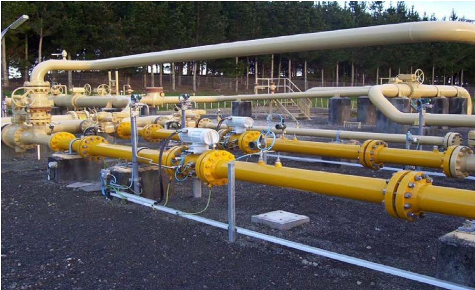
Figure 4 - two ultrasonic meter streams
