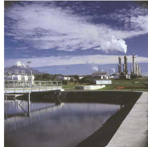
Kapuni Gas Treatment Plant
