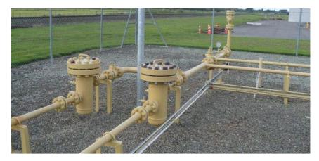
Figure 3 - Filters at the start of two metering 'streams' on a transmission system delivery point
