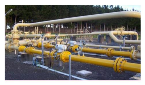
**Figure 5 - two ultrasonic meter streams** (source: First Gas, Transmission Asset Management Plan 2018, Figure 32)
