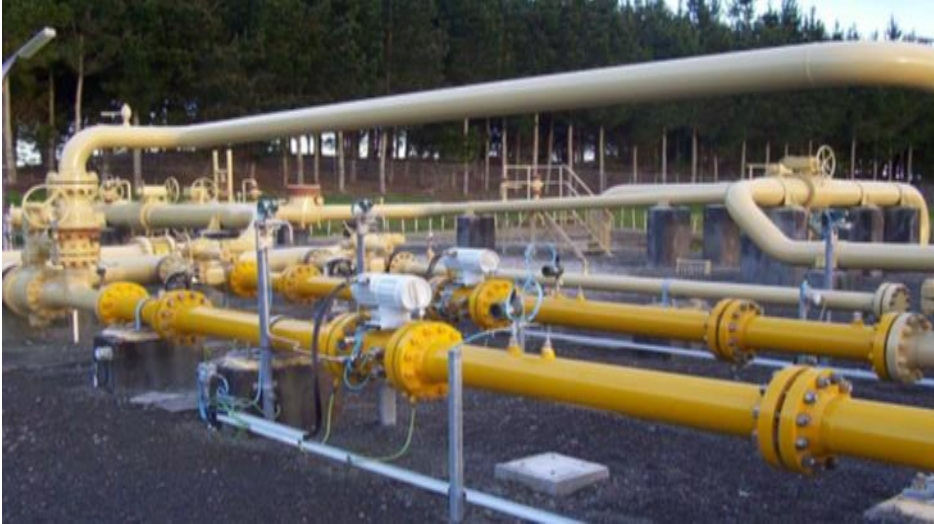
Figure 5 - two ultrasonic meter streams
